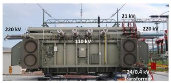
Figure 1 View of the 300 MVA Transformer
