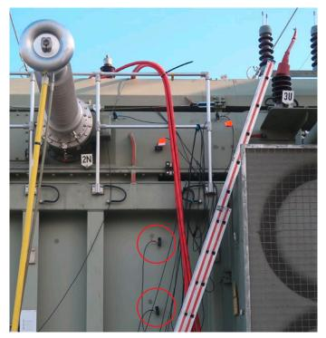
Figure 8 Installation of piezo sensors
